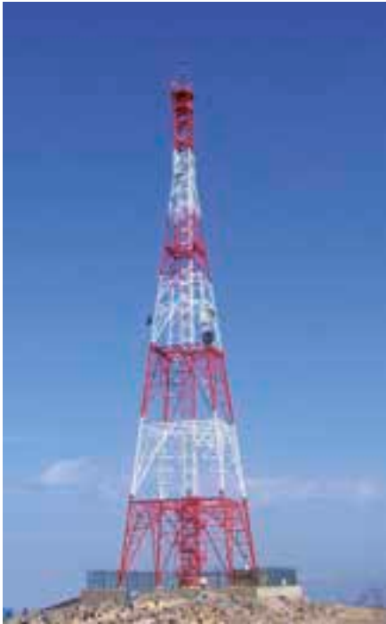
Mast with DF and monitoring antennas and a DF receiver accommodated in an all-weather cabinet on the upper platform.
