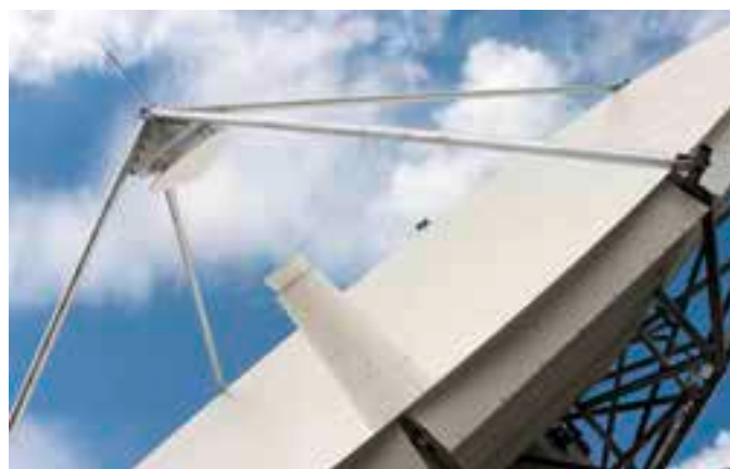
9.5 m C-band antenna installed at Munich site.
